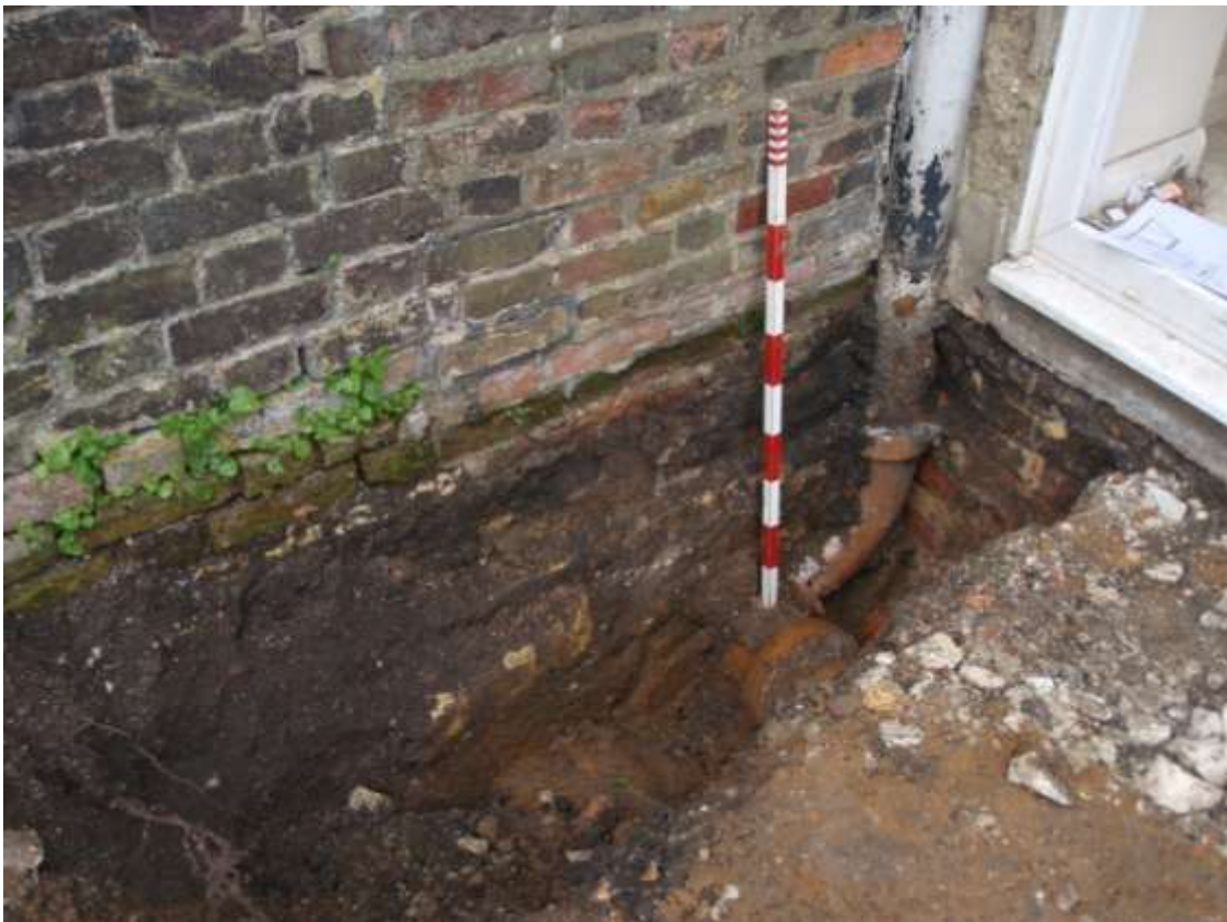
Plate 5. Exposing existing drain
