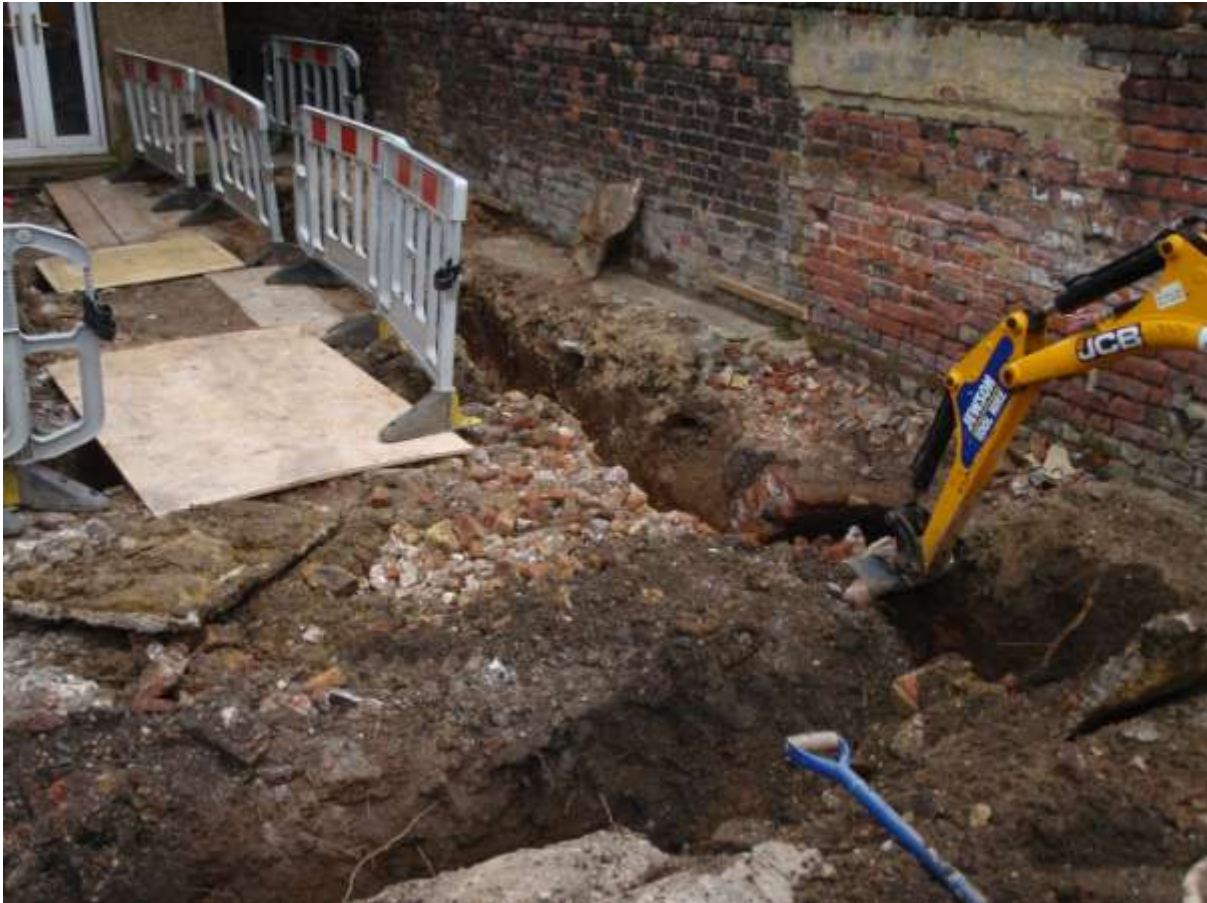
Plate 6. Cutting of the foundation trenches on west side and brick septic tank (looking south)
