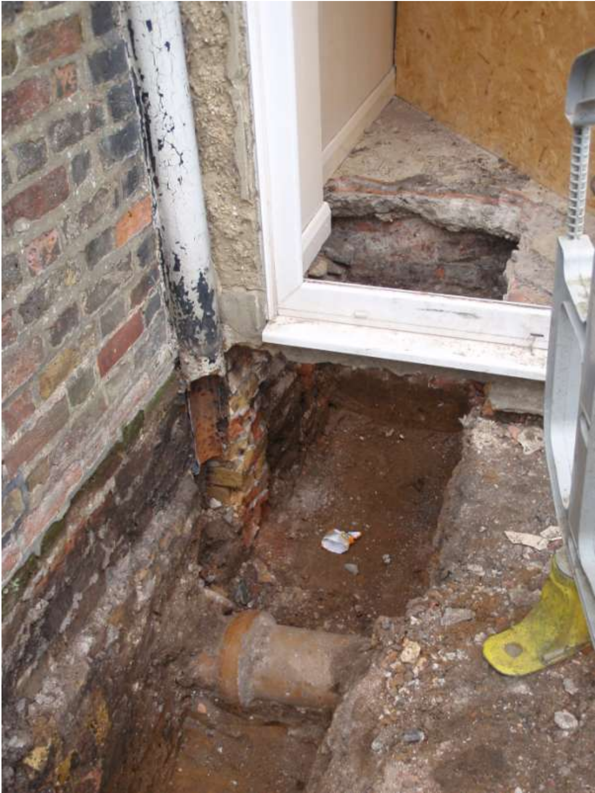
Plate 5. View of the existing drainage connection (looking south-east)
