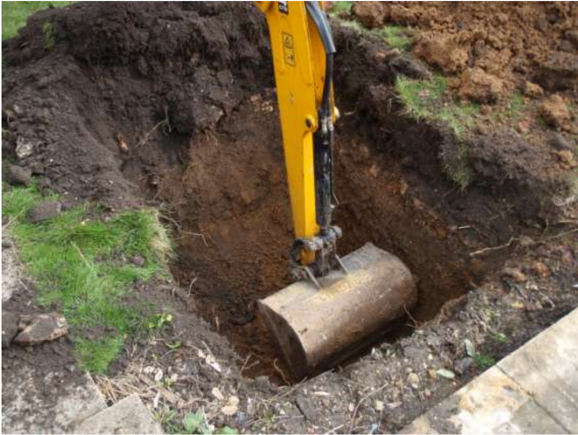
Plate 4. View of the trench (looking north-east)
