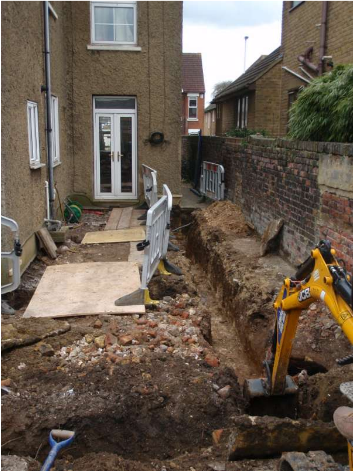
Plate 9. Foundation trenches completed (looking south)
