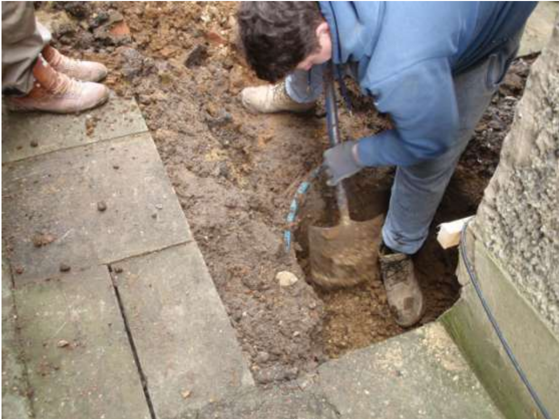
Plate 2. View of initial excavation of services
