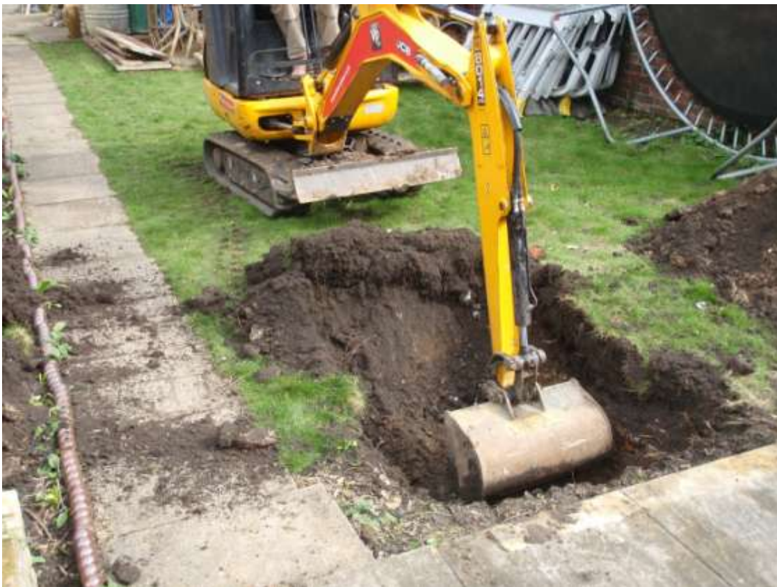
Plate 3. View of the site being tested for services (looking north-east)
