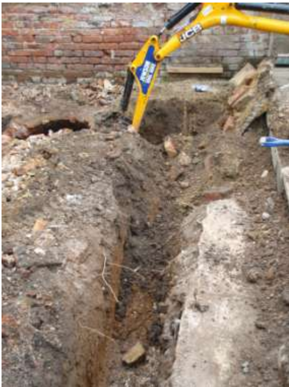
Plate 7. View of south-west trenches (looking west)
